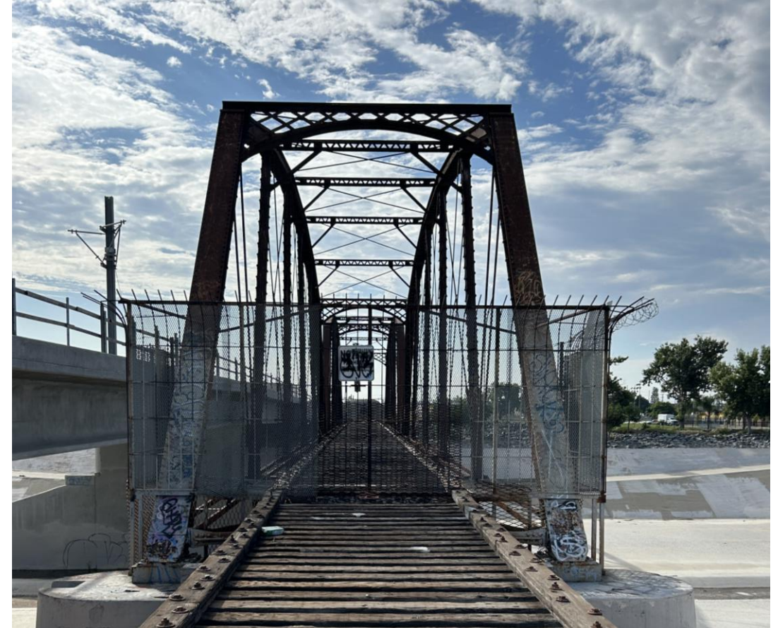
Historic PE ROW Bridge across the Santa Ana River
