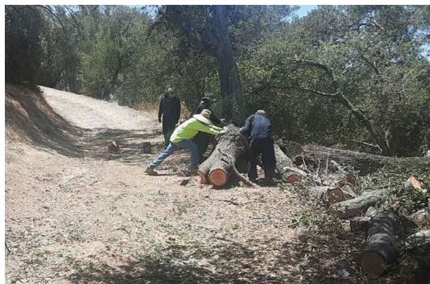
Workers manually removing fallen oak tree debris from the fire road.
