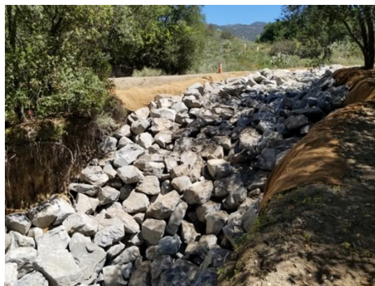
Phase 1 gully repair project near entrance of Trabuco Rose.
