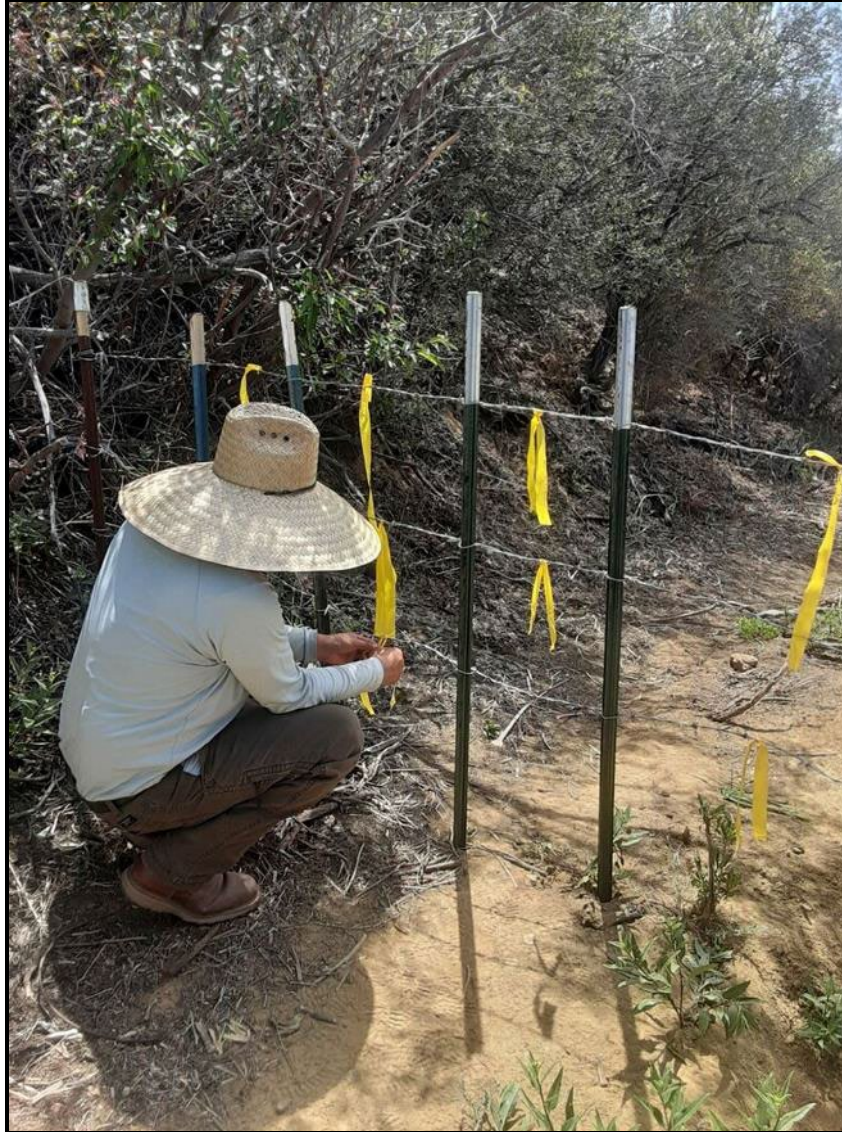
PHOTOGRAPH 19 Additional Posts and Flagging Added to Damaged Fence, Silverado Chaparral Preserve, May 2021
