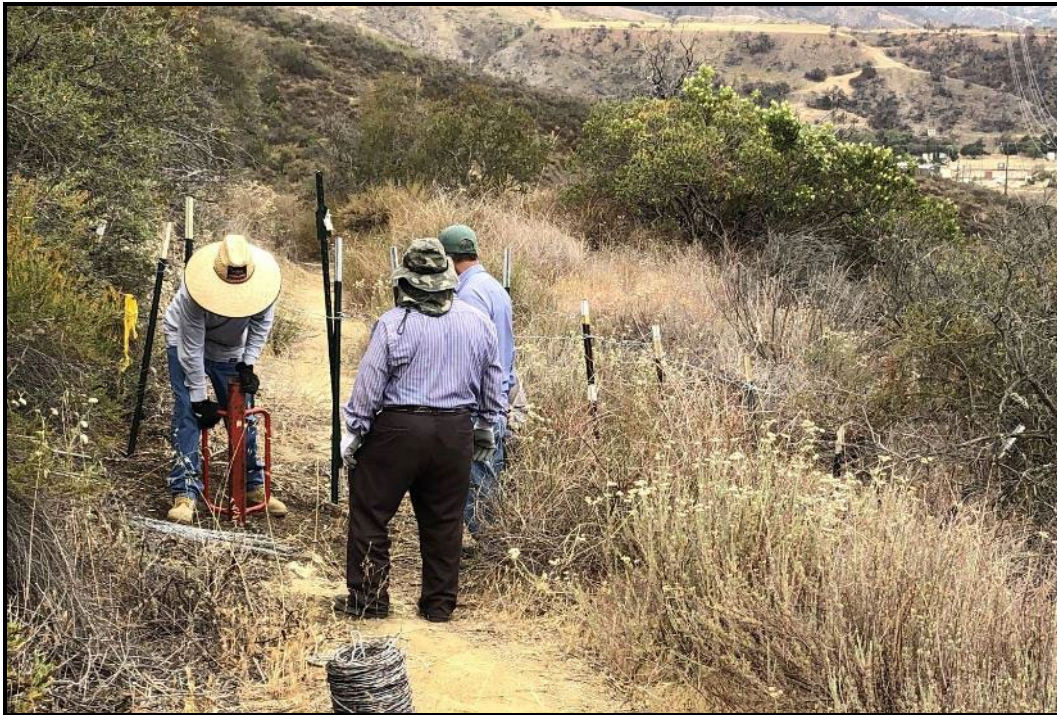
PHOTOGRAPH 21 Fence Repairs to Deter Unauthorized Access, Silverado Chaparral Preserve, June 2021
