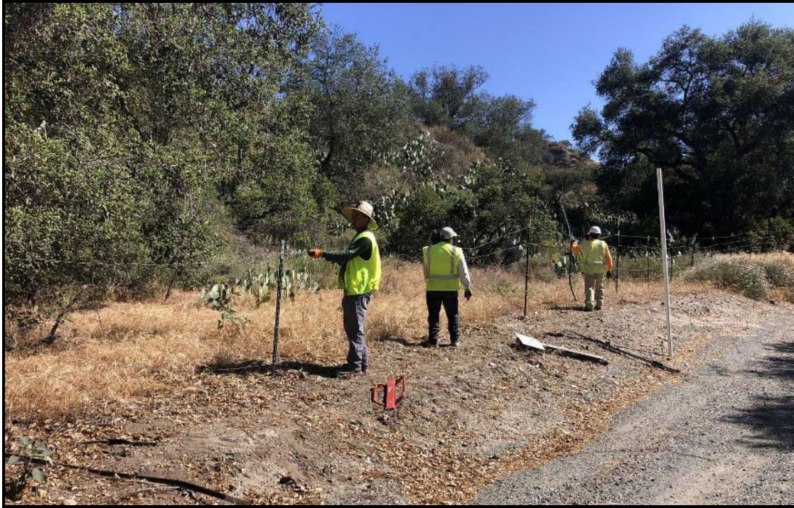
PHOTOGRAPH 13 Fence Repairs Along Trabuco Canyon Road, Wren's View Preserve, May 2021
