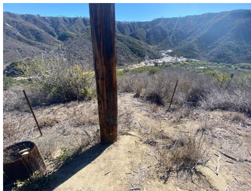
Area cleared of vegetation by SCE around a power pole.
