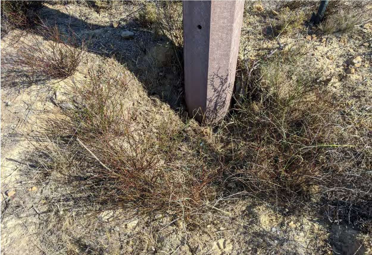
4633687E After Photos – kikuyu grass and red bromes manually removed around the pole
