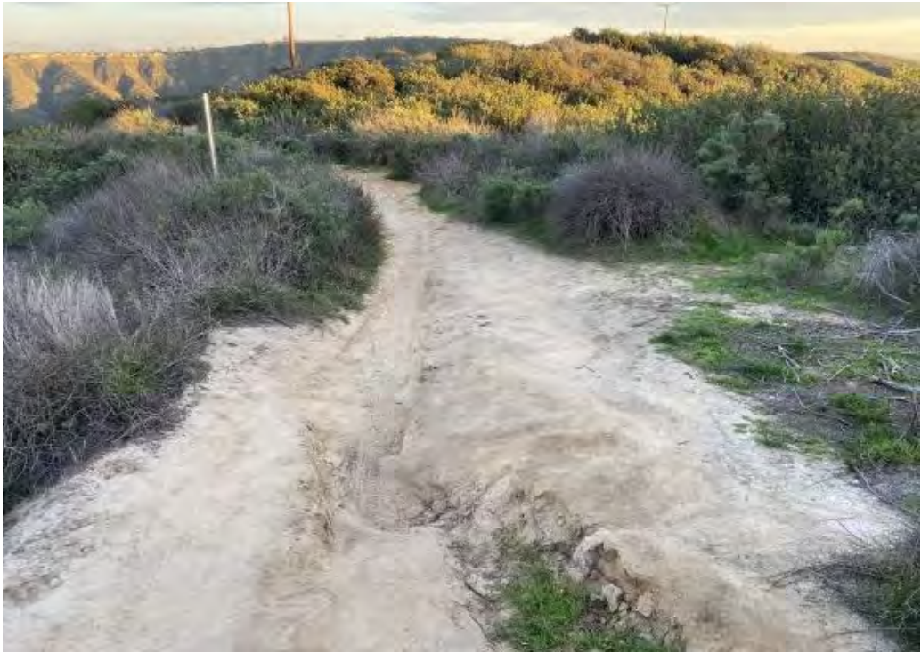
Photograph 8: View of area that may need additional recontouring. Photo dated January 26, 2022.
