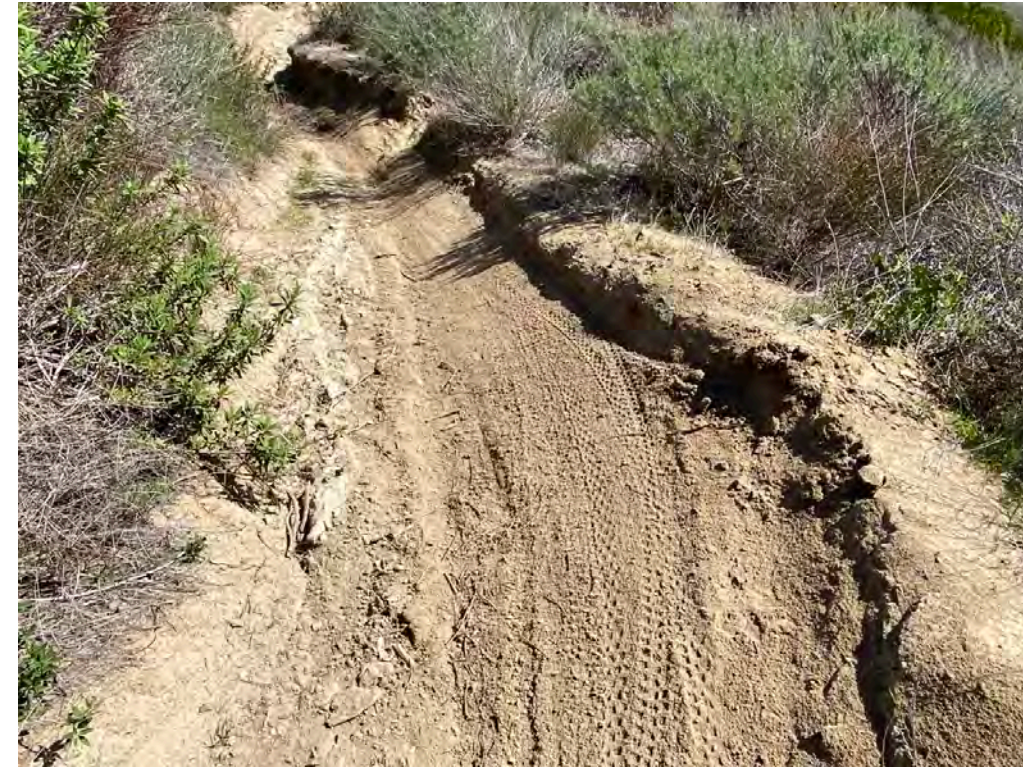
Photograph 2: View of mountain bike tracks and severe erosion on "Kamikaze Trail" facing east. Photo taken October 12, 2021.
