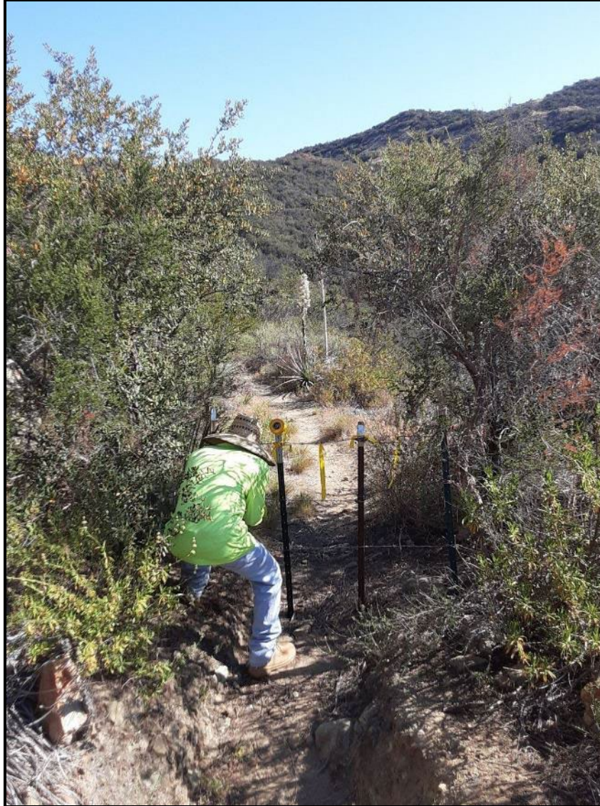
PHOTOGRAPH 18 Fence Repairs to Deter Unauthorized Access, Silverado Chaparral Preserve, May 2021
