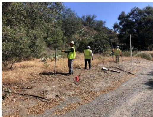
Fence line repair crews at Wren's View.
