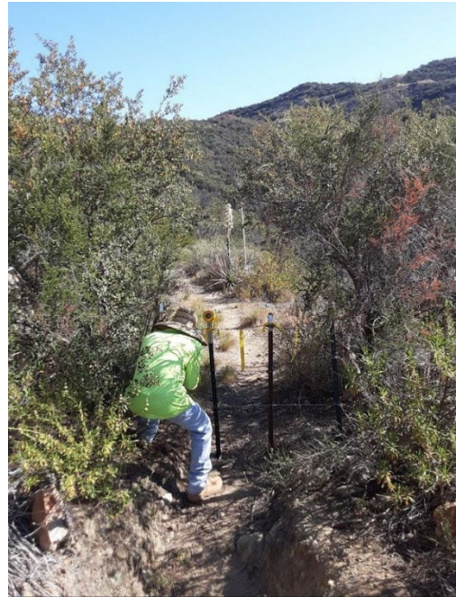
Photo of fence repairs to deter unauthorized access.
