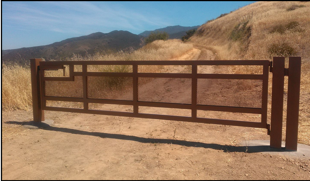
PHOTOGRAPH 19 New Gate on Fire Road at Northeastern Boundary of Silverado Chaparral Preserve, Installed in May 2022
