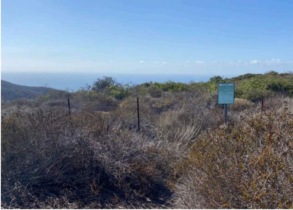
Photograph 2: View of decommissioned trail and previously repaired fencing and added signage. No signs of recent bike or pedestrian disturbance in the decommissioned area. Lower left-hand side views treated iceplant. Photo dated October 27, 2022.
