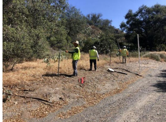
Fence line repair crews at Wren's View.
