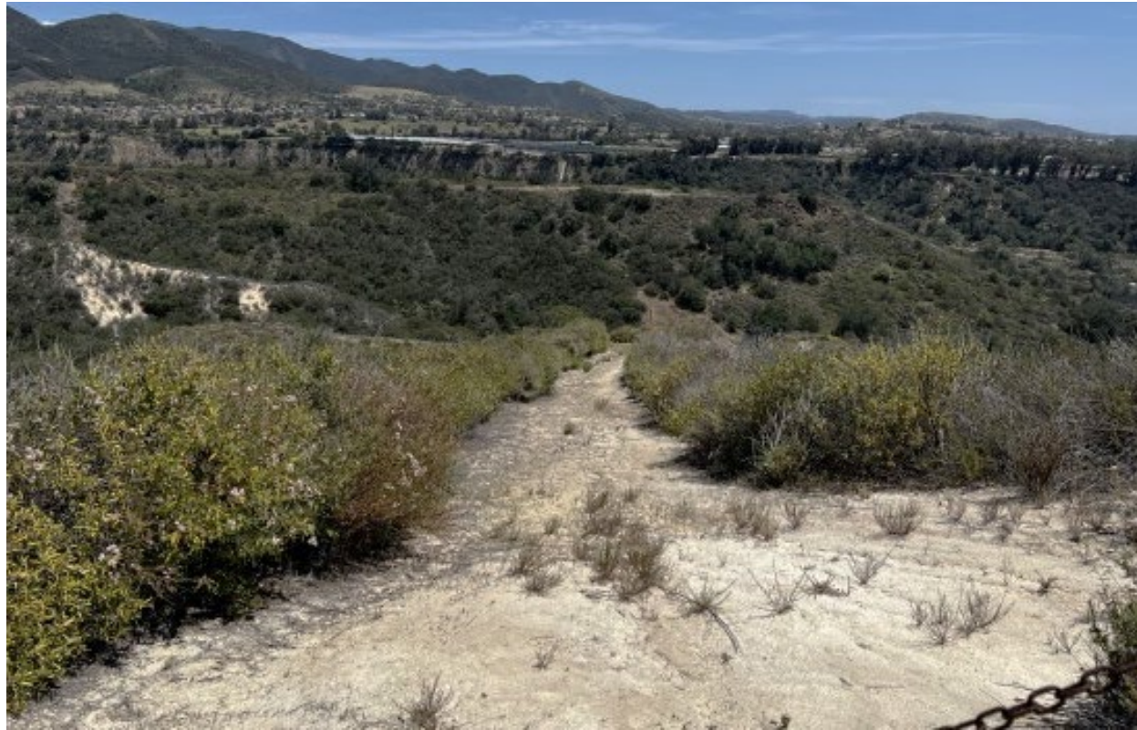
Photograph 9: View of Trail 9. Conditions remain consistent with previous years. No active restoration is recommended. Continue to monitor for invasive species.
