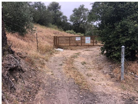
Photo of the new gate installed. Photo courtesy of RECON.
