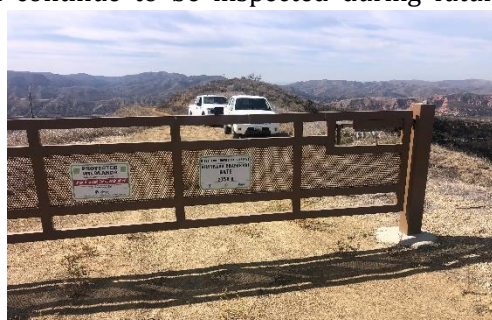
New gate installed to help minimize illegal access at Silverado Chaparral Preserve. Photo courtesy of RECON.
