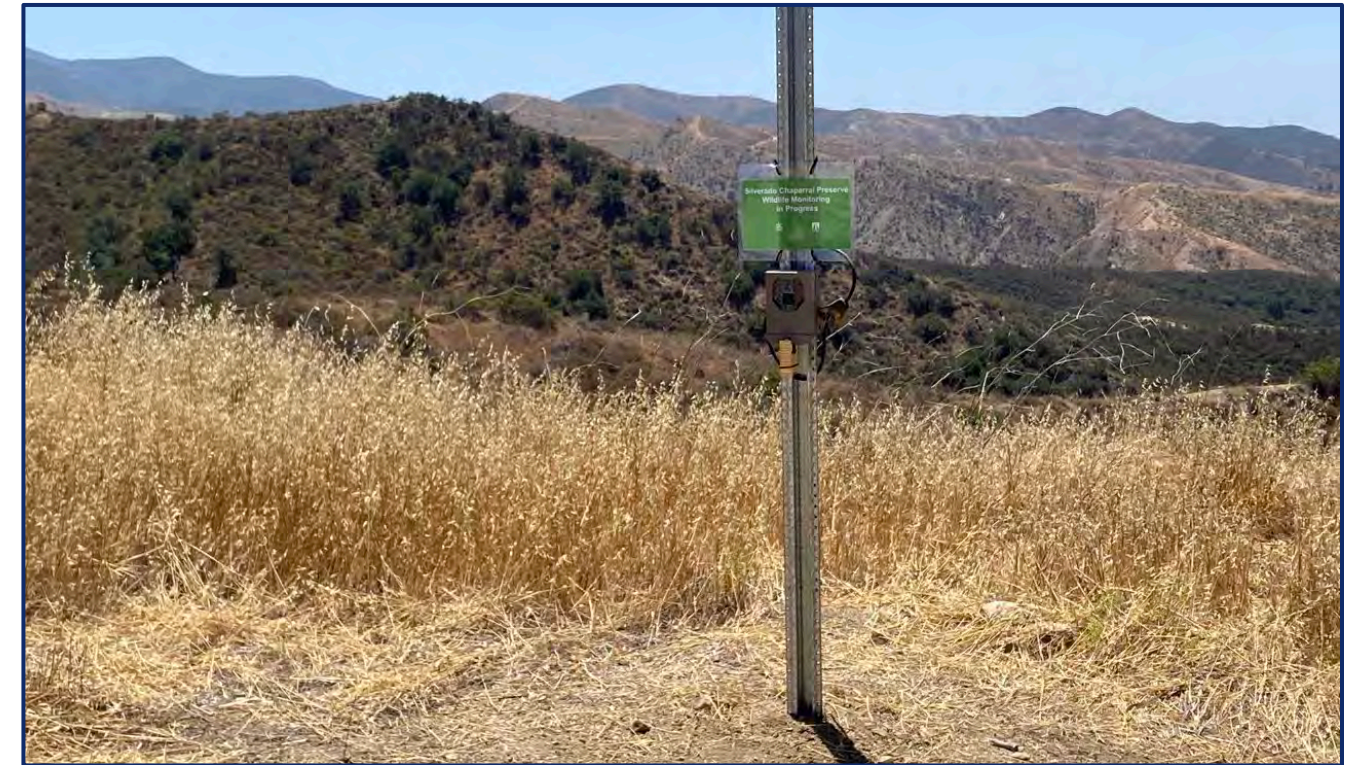
Photograph 2: View of installed wildlife camera A. Photo taken June 14, 2022.
