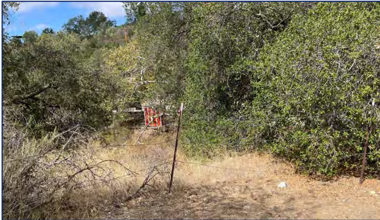
Photograph 11: Depicting area in need of fence repair. Photo taken September 14, 2022.
