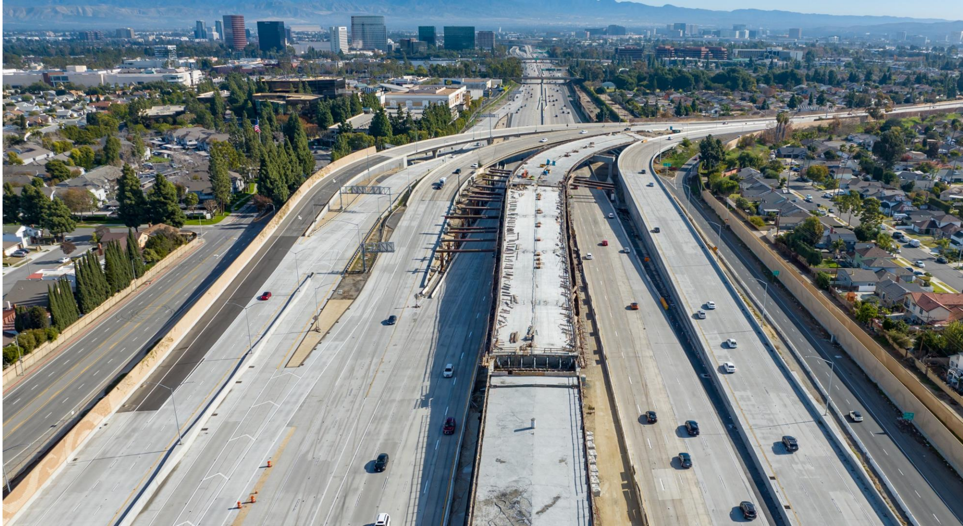
I-405/State Route 73 (SR-73) median connector bridge construction
