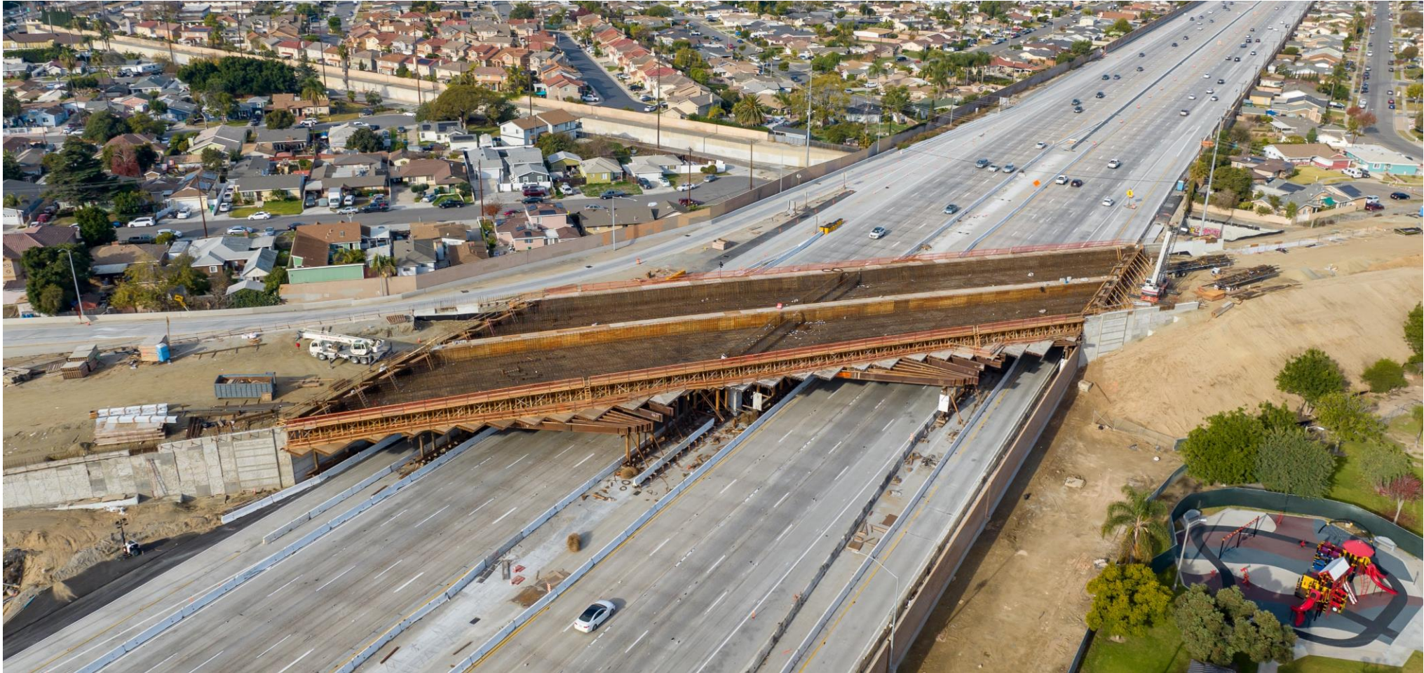
Springdale Street bridge construction
