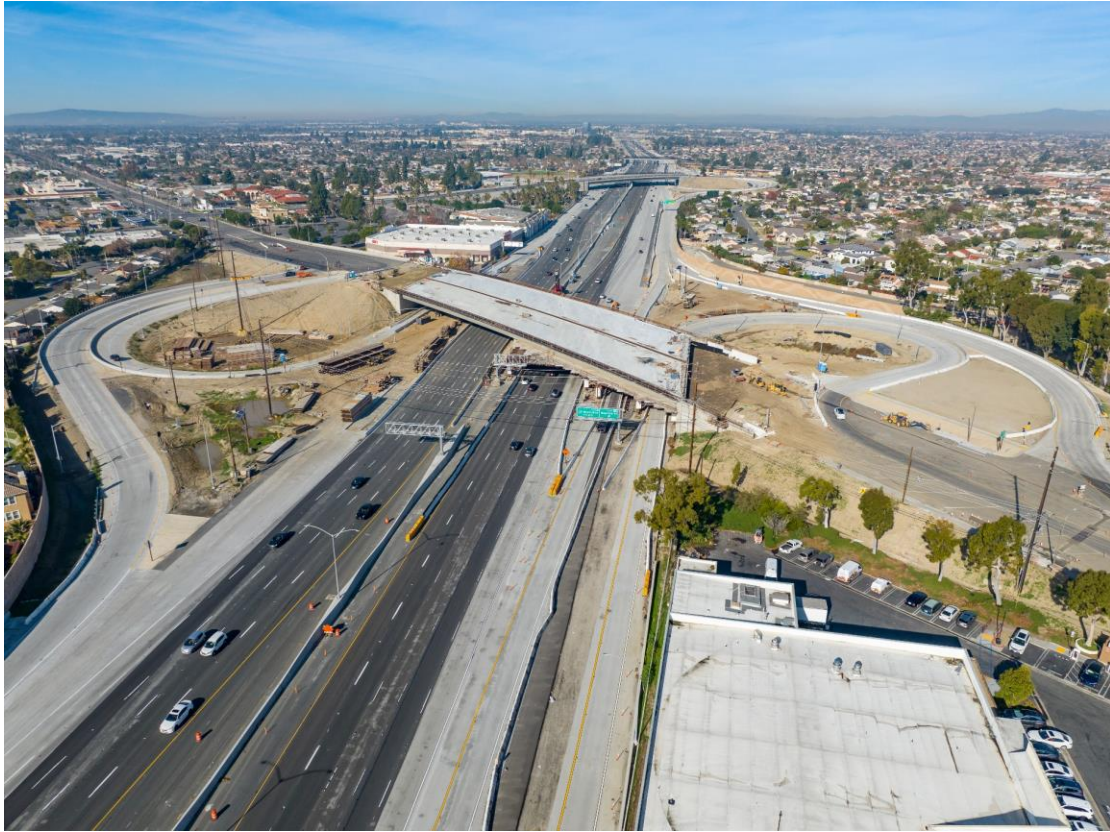
Warner Avenue bridge construction
