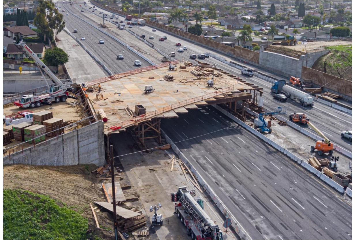
Newland Street bridge construction
