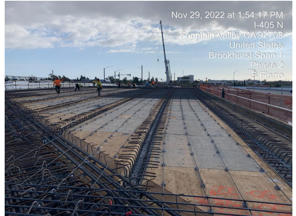
Brookhurst Street bridge construction
