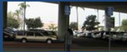
Old Town Station
